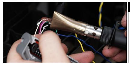
Ensure the CAN splices are sealed against water ingress.
